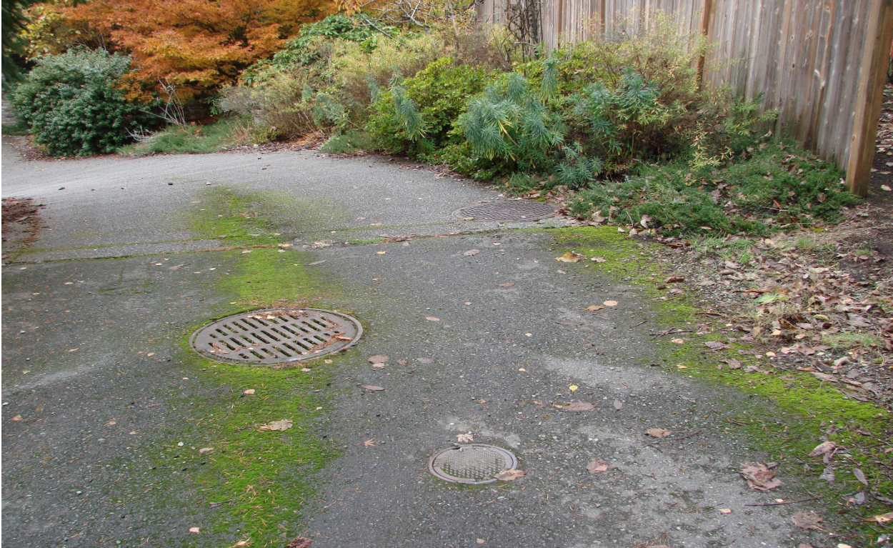
Photo #8 – West end of shared access – CB#22-168 (with solid round lid)
