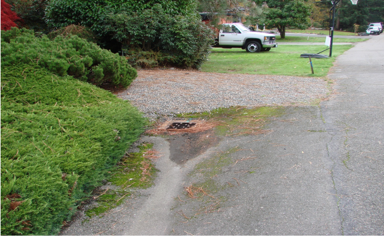
Photo #4 – View south on 83 rd at Cb#22-111
